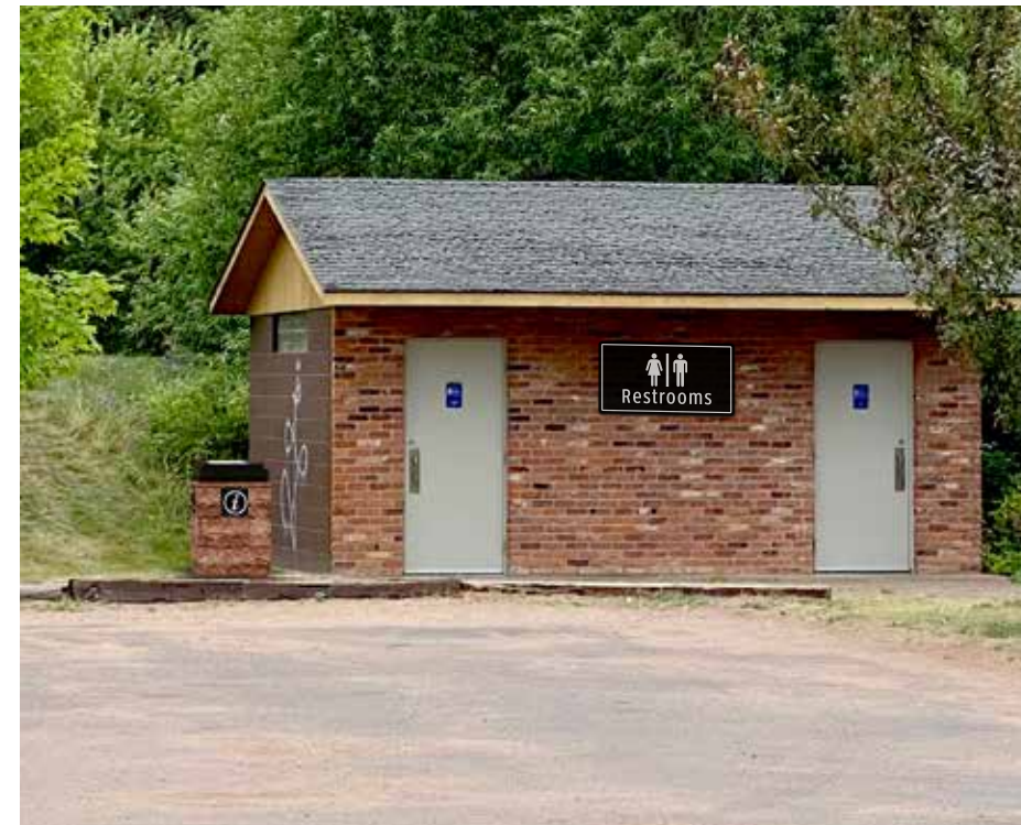
5 Photo Composite SCALE: NTS Washington St Restrooms
