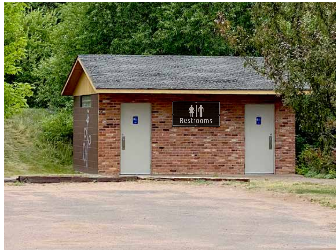
4 Photo Composite SCALE: NTS Washington St Restrooms
